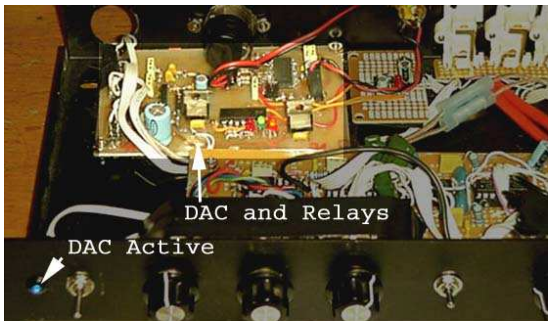
Photo of DAC Unit
